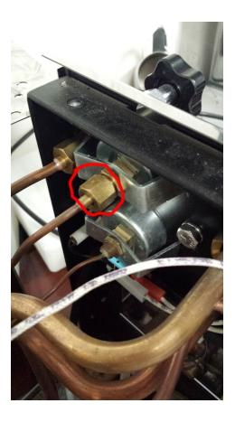
Once that nut has been loosened and moved back, you will need to undo the smaller nut in front of that shown (circled in red).
